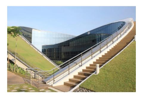
Another alternative to traditional roofing materials is a rooftop garden or **"green roof**." Green roofs replace heat-absorbing surfaces with plants, shrubs, and small trees that cool the air through **evapotranspiration**.
