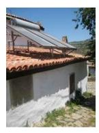
**Heating Water:** Homes can use passive solar heating to provide hot water for showers and washing dishes. Thin rectangular tanks with a glass front are positioned on the roof. The water circulating through the tank is heated by the sun's energy. The system relies on gravity to deliver hot water on demand.
