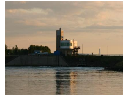
Annapolis Royal Generating Station (Canada, 1984)
