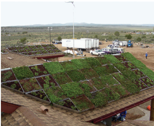
Figure 14: A Modular Green Roof on a Sloped Residential Roof
