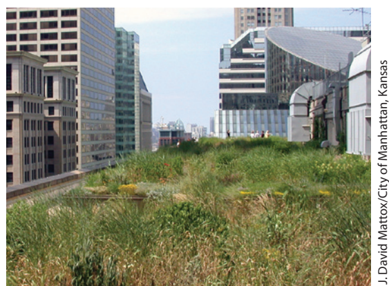
Figure 5: Combination Extensive/Intensive Green Roof—The Rooftop Garden on Chicago’s City Hall
