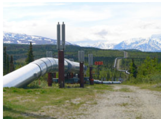
Pipeline Across Alaskan Lands
